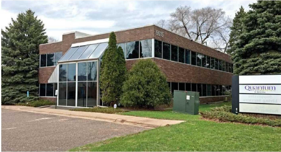
Image 1. Exterior and Interior Images of Subject Property (5615 Brooklyn Boulevard).
