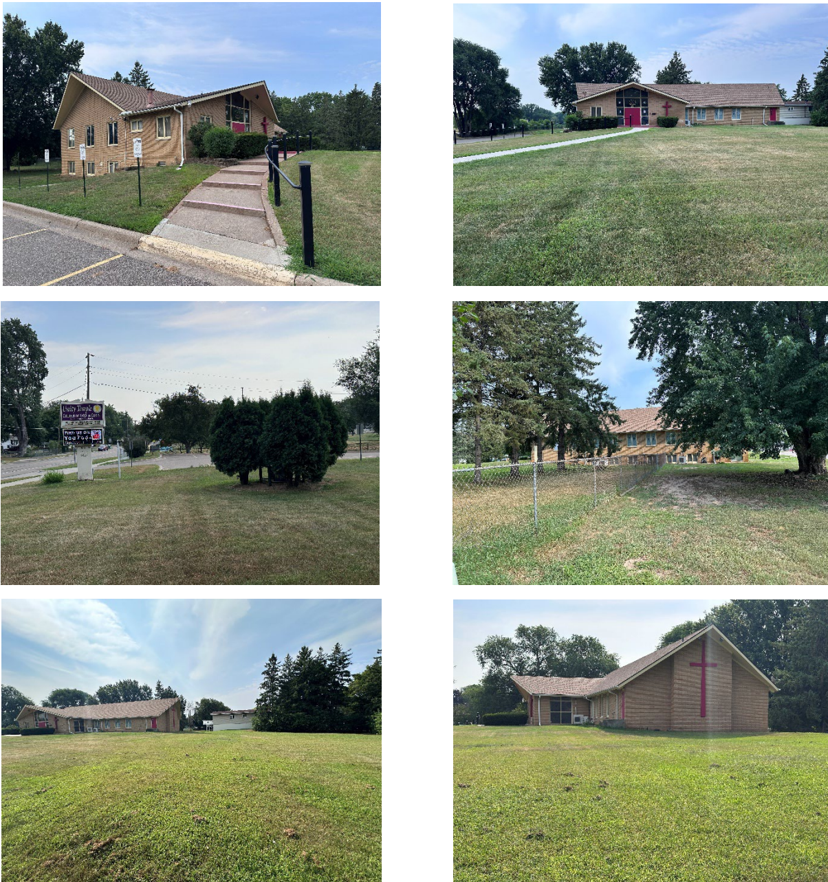
Image 1. Existing Site Conditions at Subject Property.
