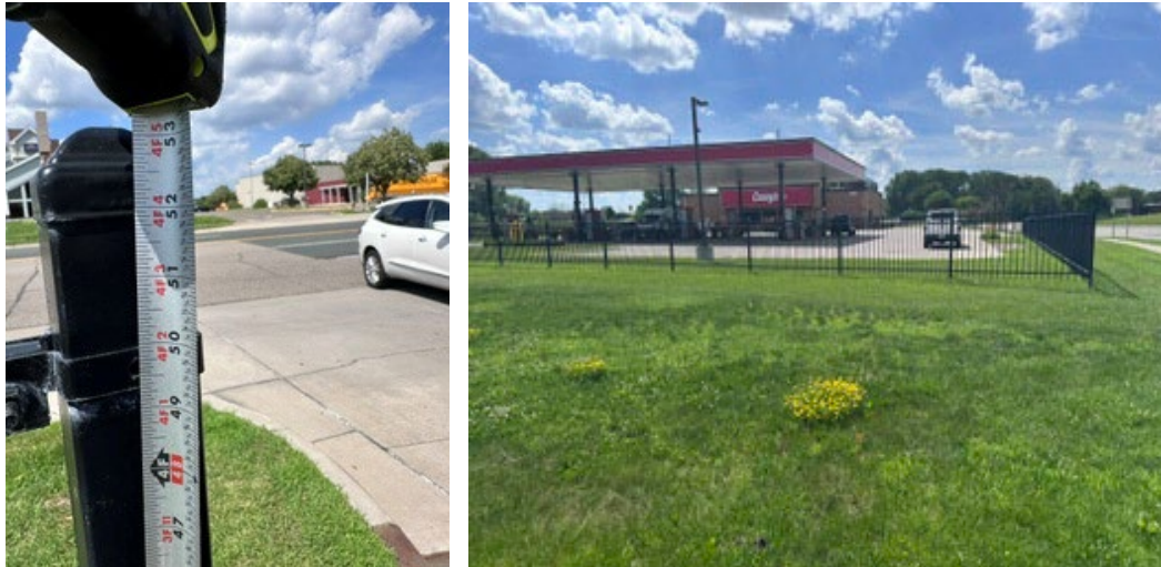
Image 2. Fence installed at Casey's Gas Station (2101 Freeway Boulevard).
