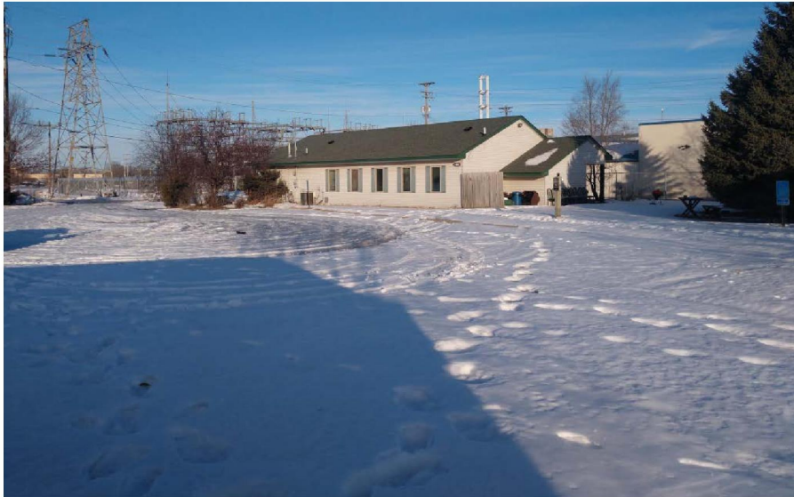
Image 2. Extent of Parking Lot—Taken from Southeast Edge of Parking Lot Adjacent to Trash Enclosure.
