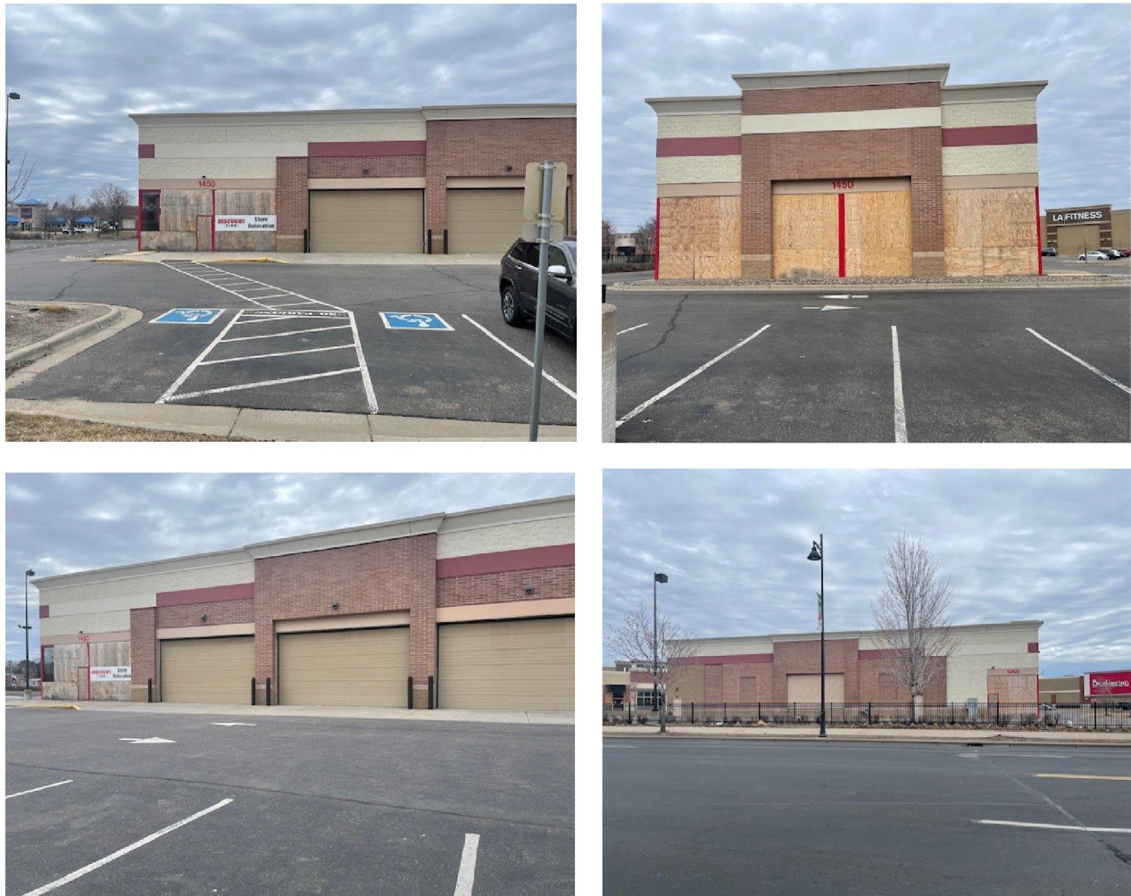
Image 1. Existing Site Conditions at Subject Property.
