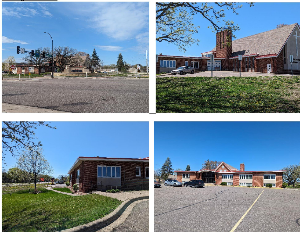
Image 1. Existing Site Conditions at Subject Property.
