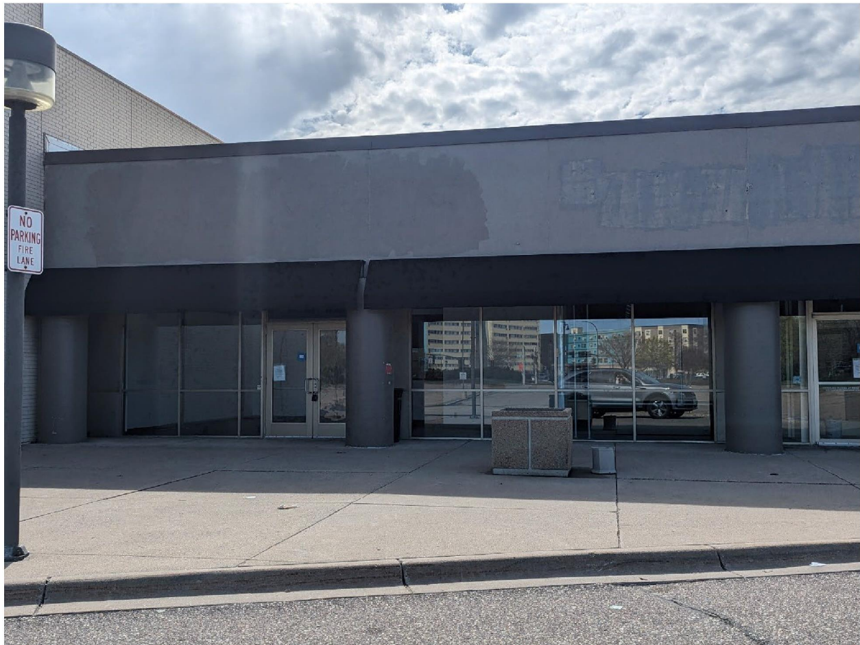
Image 1. Existing Site Conditions at Subject Property.
