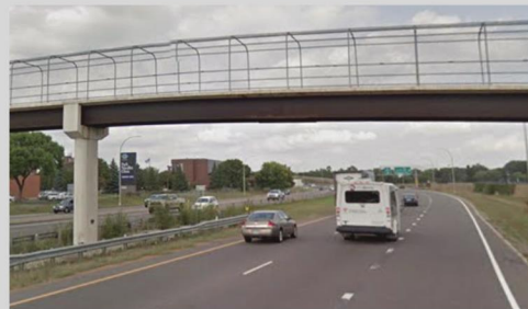
Pedestrian Bridge over Hwy 100
