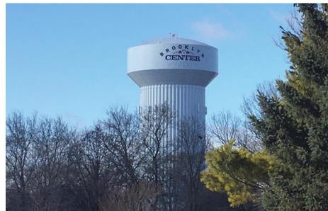
Brooklyn Center Water Tower
